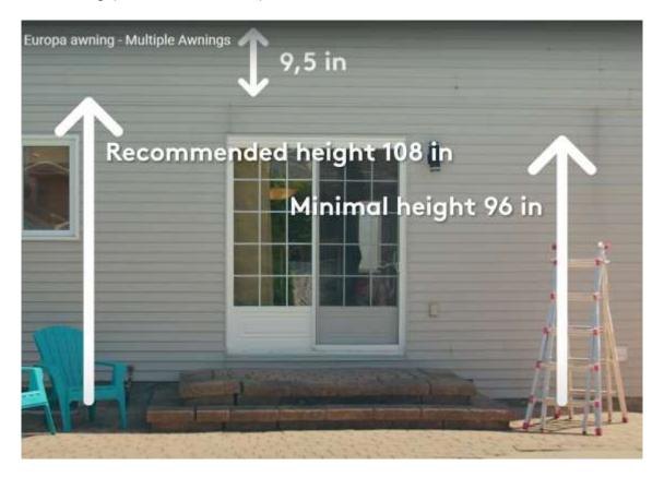
If your awning is motorized, it must be plugged into a GFI electrical outlet. The motor's electrical cord is 24' long. The motor's amperage requirement is fewer than 2 amps (2A).
